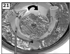
Install light fixture by twisting plate with key hole slots into place. Replace screw removed and tighten the 3 screws securely.
